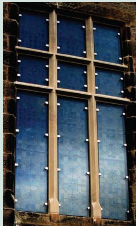
The completed work from the exterior
